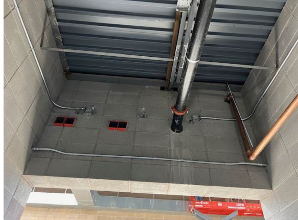
Fire Suppression & Electrical Rough-In
