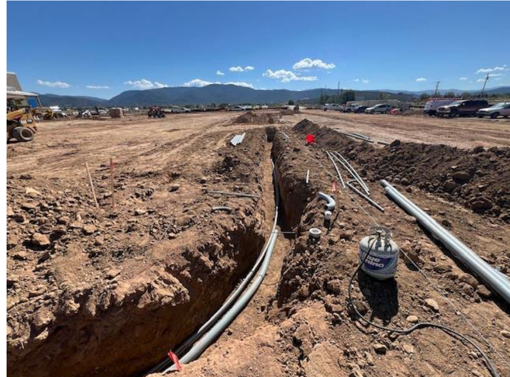
Electrical Trench for Charging Stations
