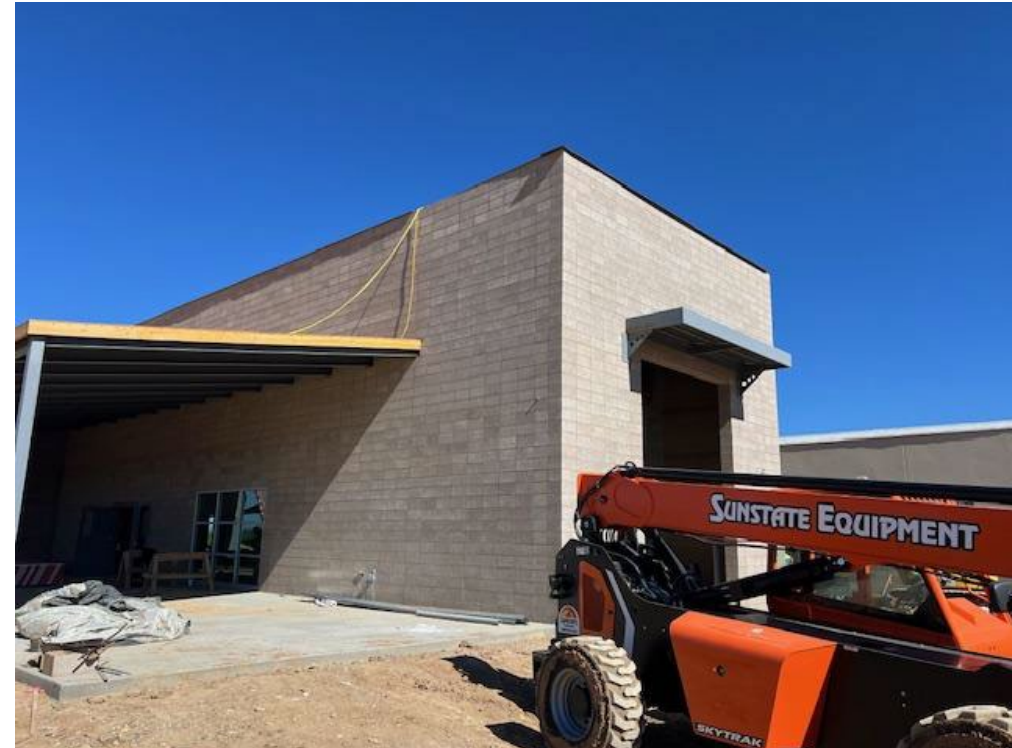
Metal Awning Installed on Wash Bay
