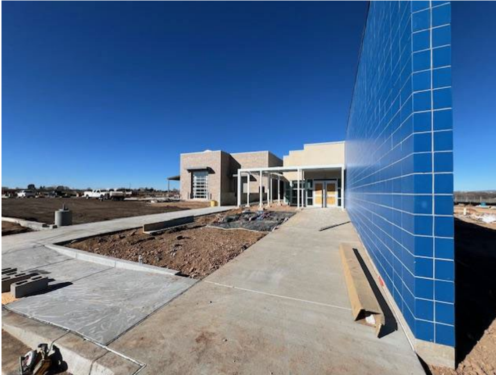
Concrete Curb and Sidewalk, Canopy Structure
