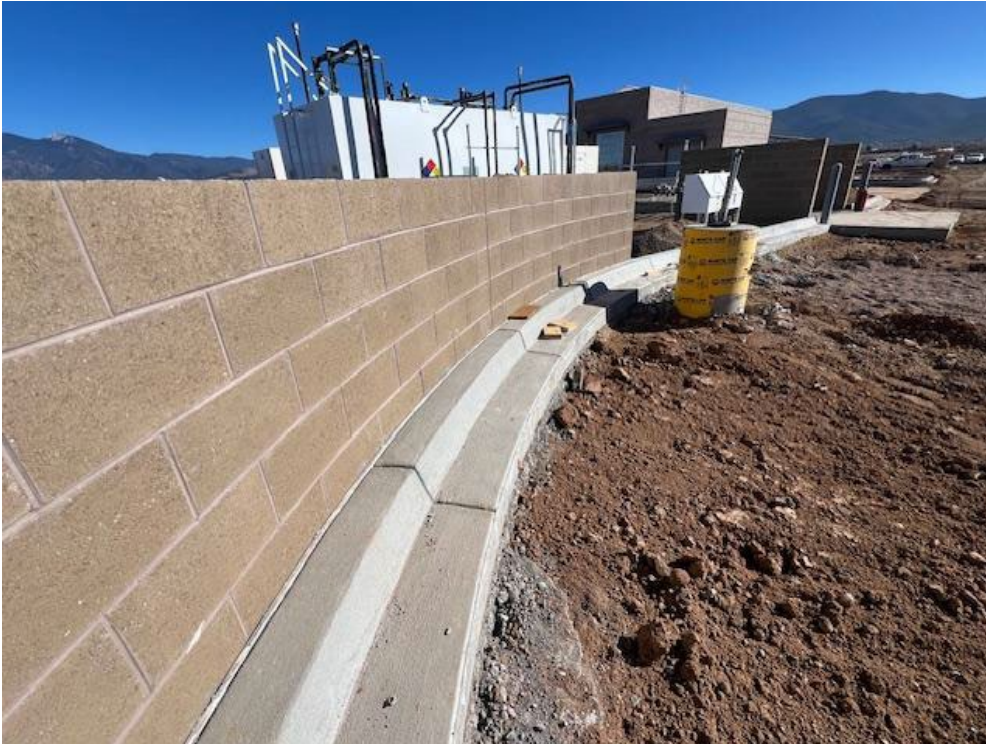
Curb and Gutter at Fueling Island Retaining Wall
