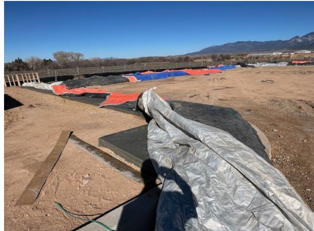
Concrete Curb, Gutter and Sidewalk Covering
