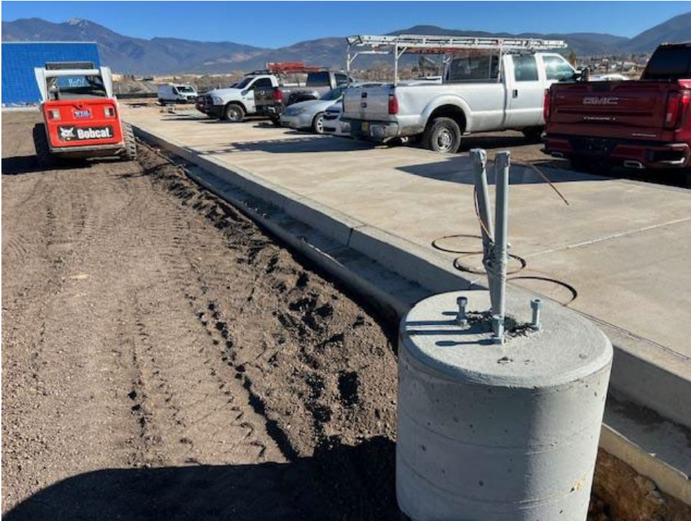
Concrete Curb, Gutter and Sidewalk, Light Pole Base
