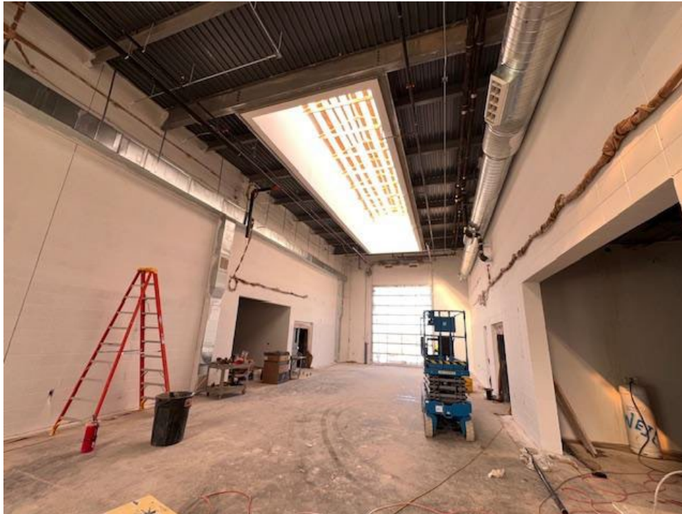
Paint, Fire Suppression System and Mechanical/Electrical/Plumbing in Service Bay
