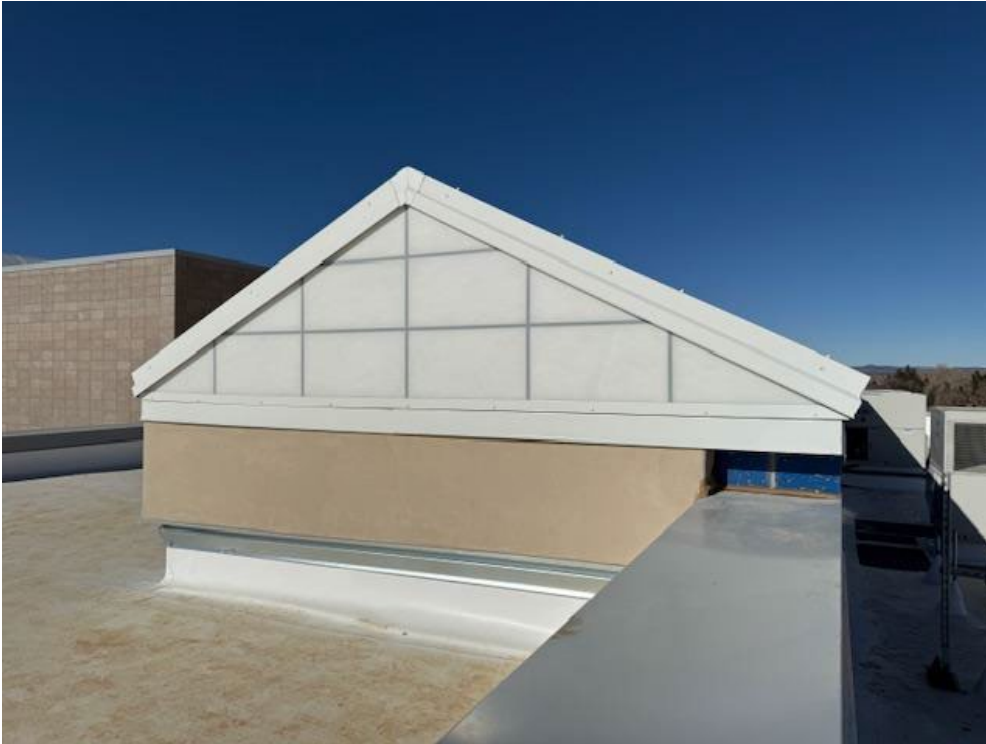
Skylight Structure & Parapet Cap
