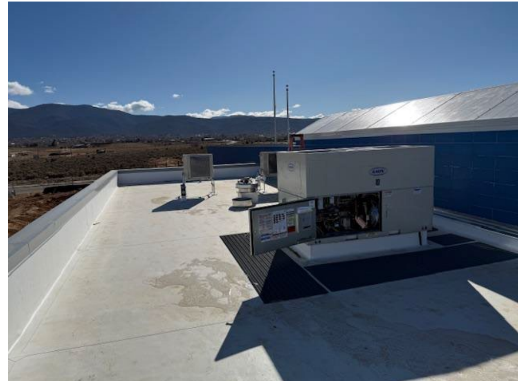
TPO Roofing * Walk Pads
