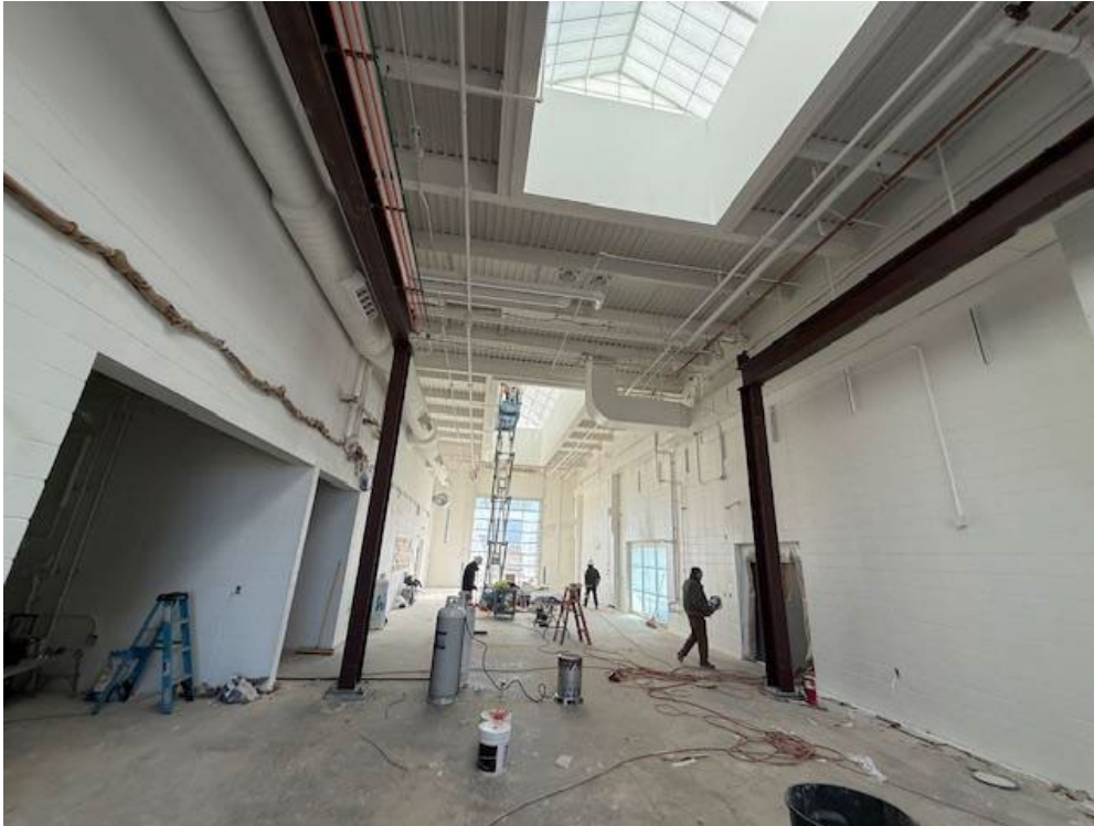
Bus Bay Bridge Crane Structure / Painting
