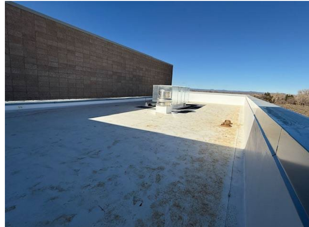
TPO Roofing & Roof Drains
