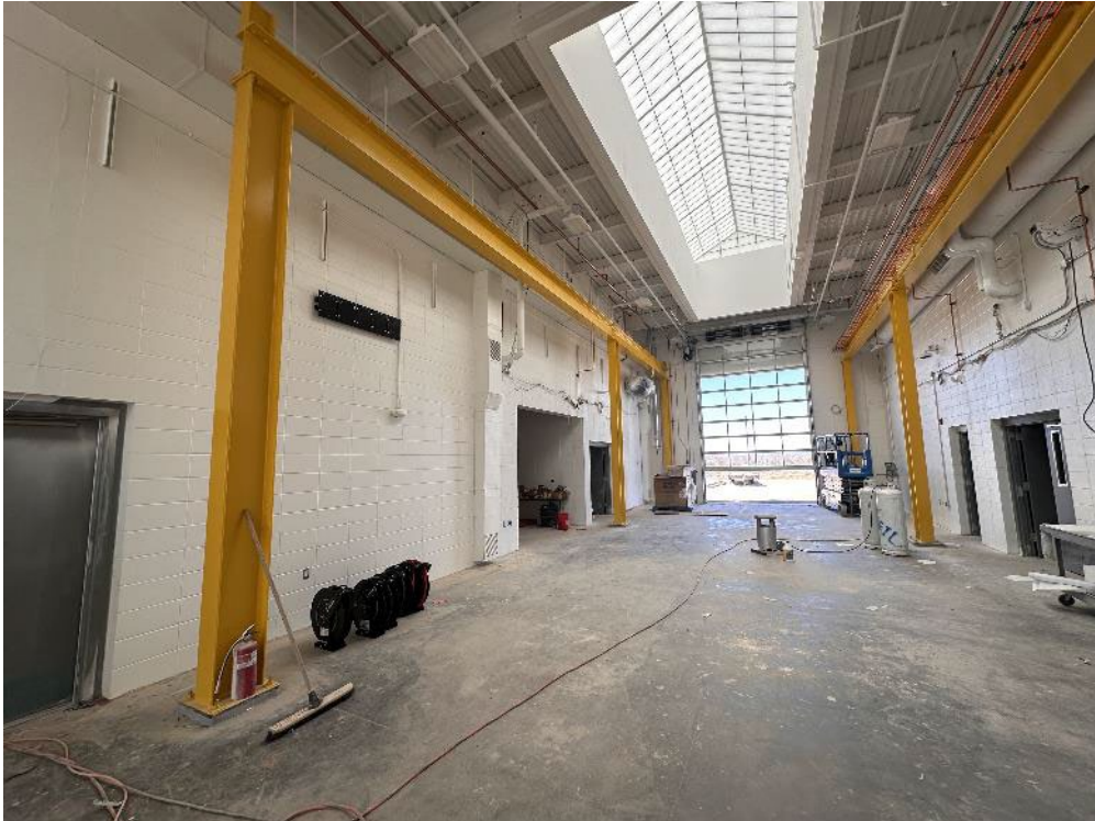
Overhead Crane Racks and Skylights
