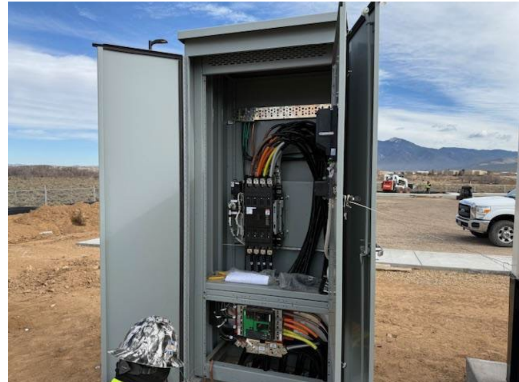
Automatic Transfer Switch Cabinet
