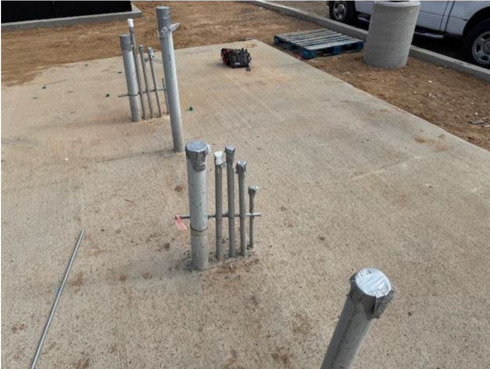
Concrete Pad and Conduit for Charging Station
