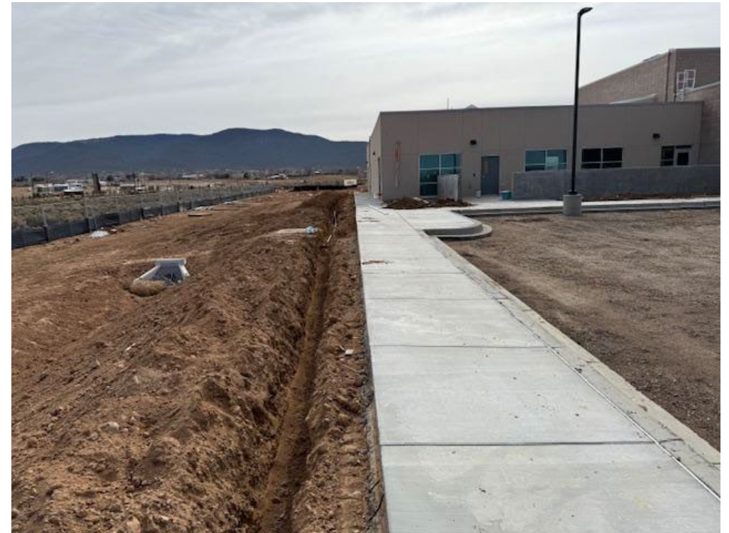
Sidewalk Irrigation Line Trench
