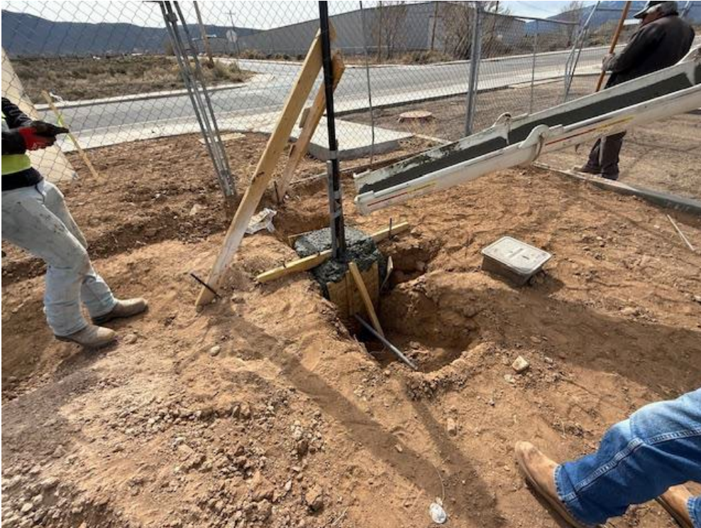
Concrete Pad for Gate Sensor at Bus Entrance
