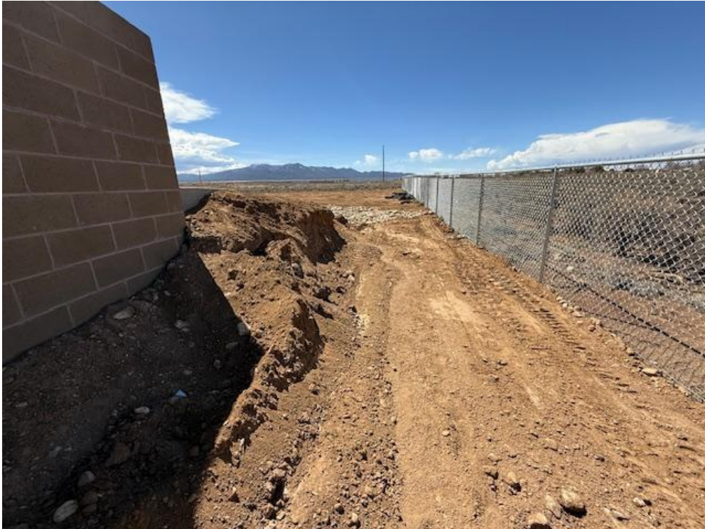
Grading at North Retaining Wall
