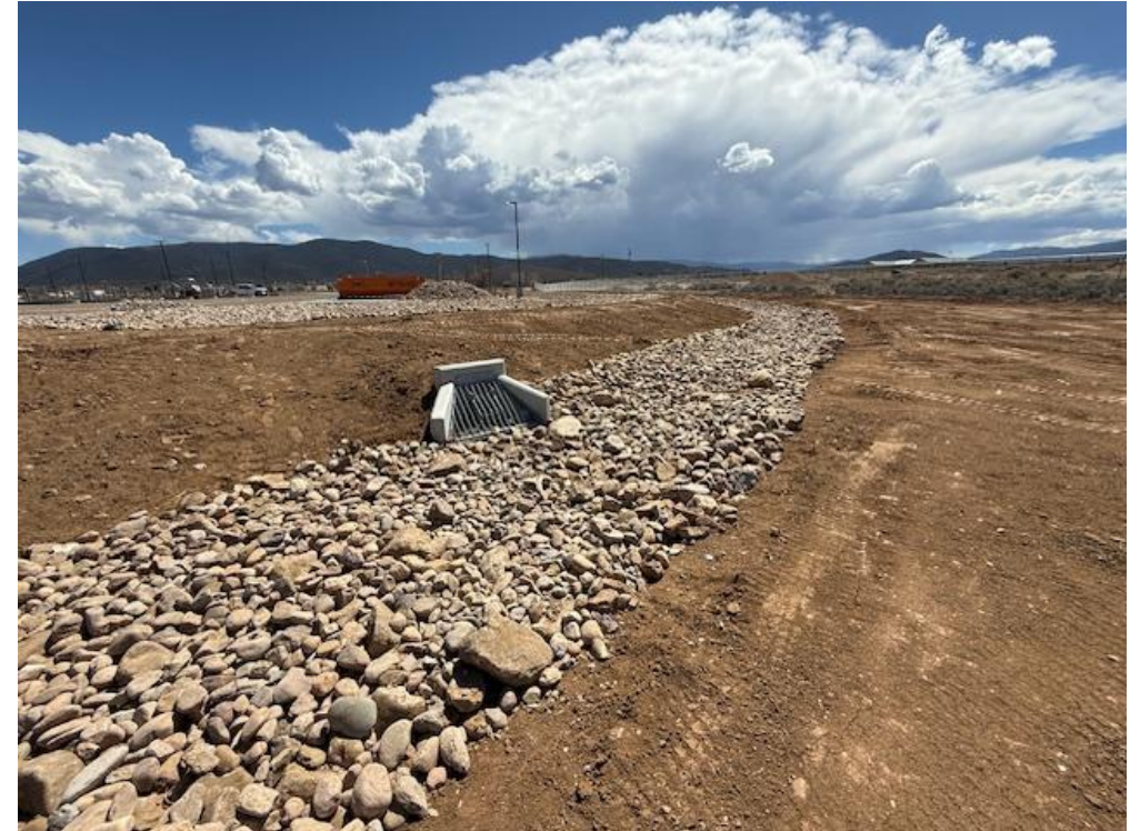
Drainage Culvert
