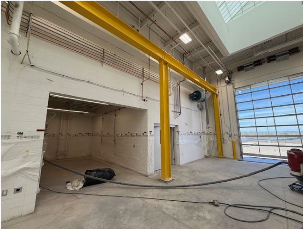
Crane Beam and Air Compressor Lines
