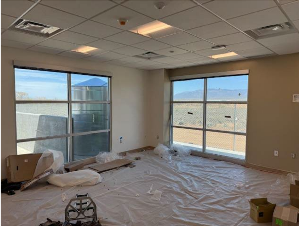
Ceiling Grid Panels and Painting
