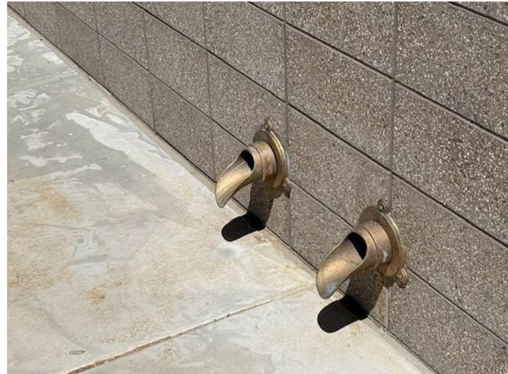
Drainage “Cow Tongue” Outlets
